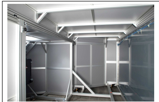
Inside the VisWall projection room, built using aluminium profiles from the item MB Building Kit System. (Left: Projector with slot-in function. Right: Projection surface)
